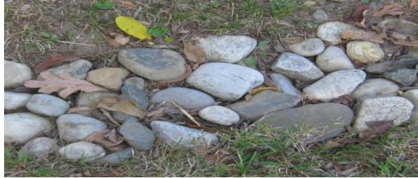
Example of a river stone overflow channel from a rain garden
