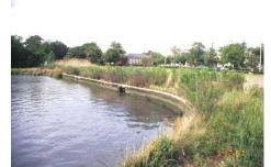
**Background**: The library's relatively protected shoreline at the dead end of a west-facing creek was lined with a concrete seawall. However, the height of the seawall did not stop periodic tidal flooding and, as a result, the library and neighboring properties supported wetland vegetation. The site also suffered from illegal vehicle abuse and neglect. The site was a former glass bottle disposal site.
