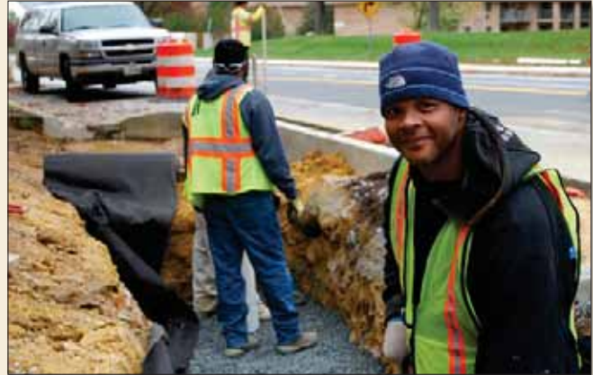
Marcus Irving, a worker at Highway and Safety Services, Inc., was unemployed before being hired to help build stormwater control systems for Montgomery County.
